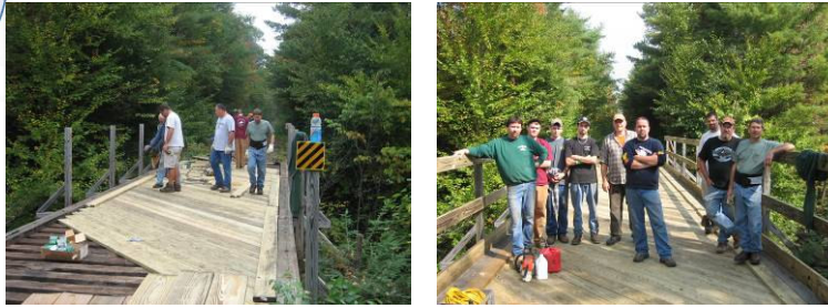
A newly decked bridge on Corridor 2
